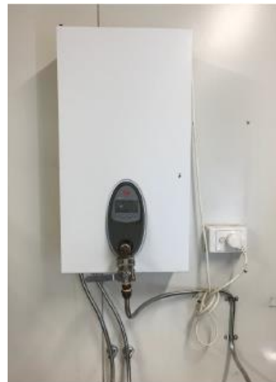
Figure 2: Existing IBW unit with on/off timer
