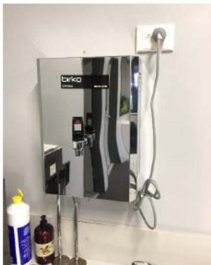
Figure 1: Existing IBW unit
