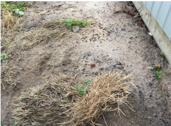
Figure 1: Underground piping running alongside shed
